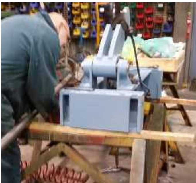
Lock and Traverse Latches for Bluescope Steel: Complete recondition including remanufacture of some parts, remachining and finally reassembly and testing.
