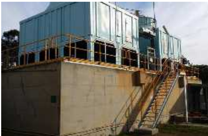
Elevated Walkways and Stairwell: Fabricated complete
